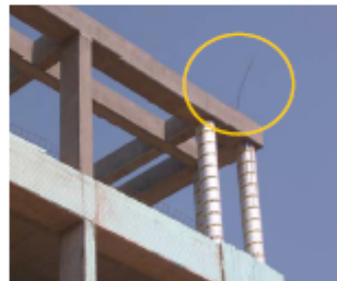
Fig 2: Down conductor installed through the reinforcement
